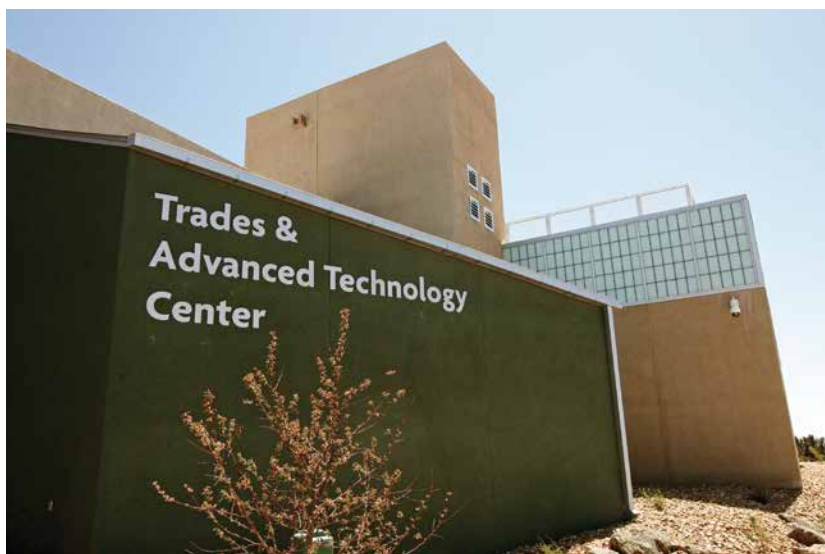
The Trades and Advanced Technology Center at SFCC
