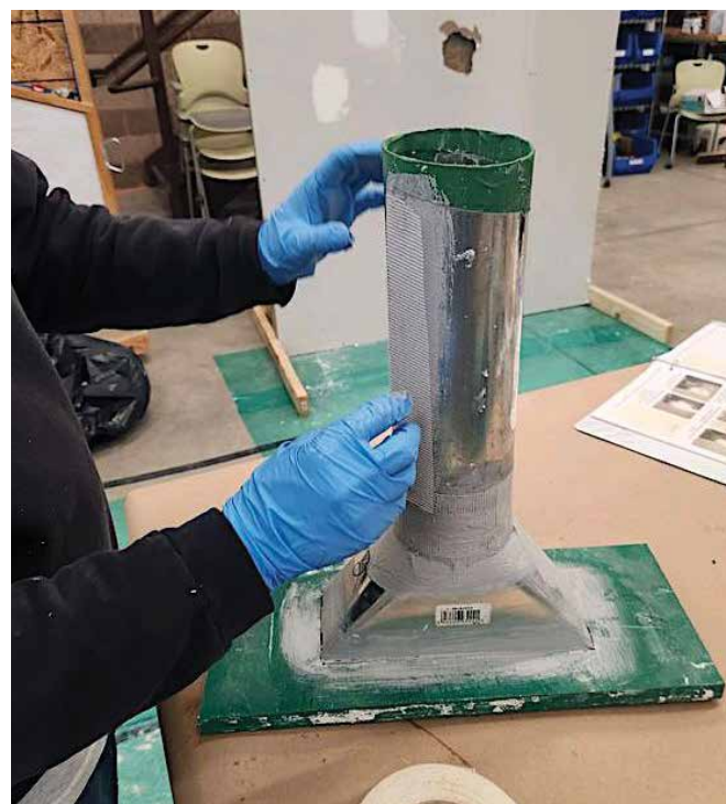
Left: The lab's test cabin; Right: a student sealing ductwork Photos © Seth Roffman and courtesy SFCC
