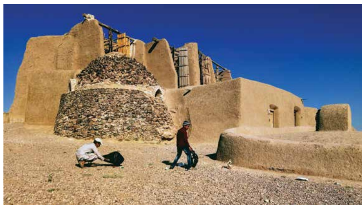
Asbads, adobe/wood vertical windmills in Iran. The windmills grind flour for the community. The bottom photo shows an ice-making and storage system that utilizes night-sky radiant cooling to produce ice, even when temperatures don't go below 40 degrees Fahrenheit. These are examples of clean, renewable energies that have been utilized for thousands of years. Photos © Alireza Khaksak
