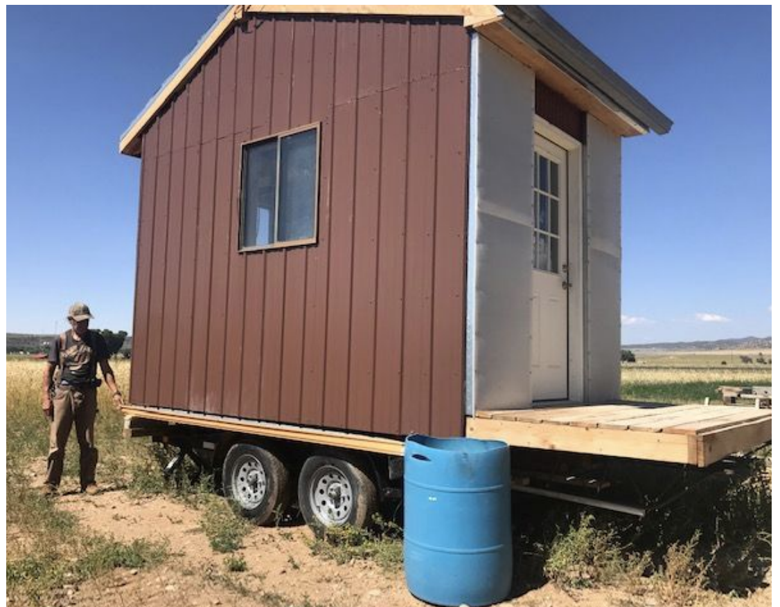
Solar cabin made of wood, hemp hurd, hempwool, etc. on a trailer
