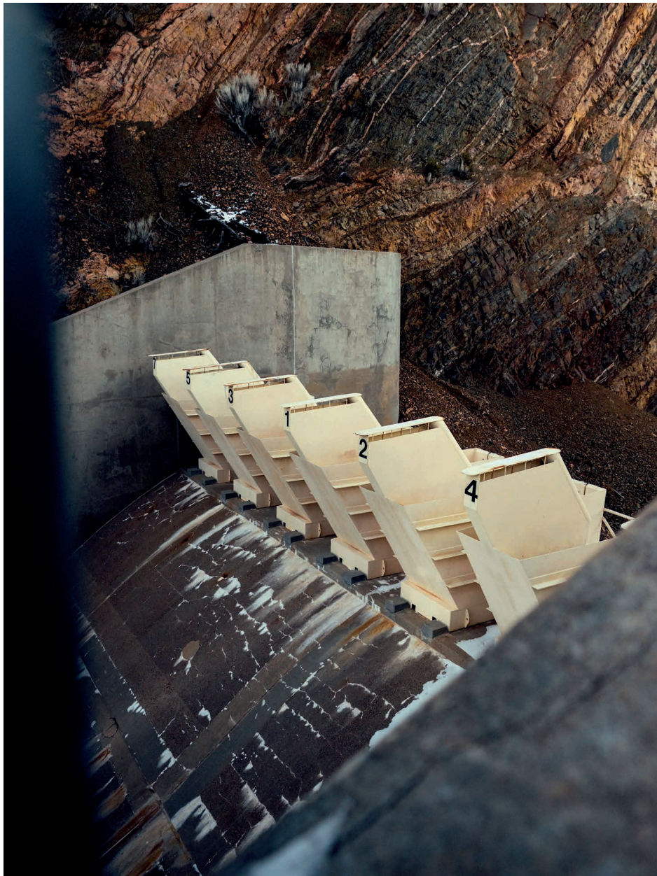
Santa Fe Reservoir Basin channel Photo by Leroy Grafe
