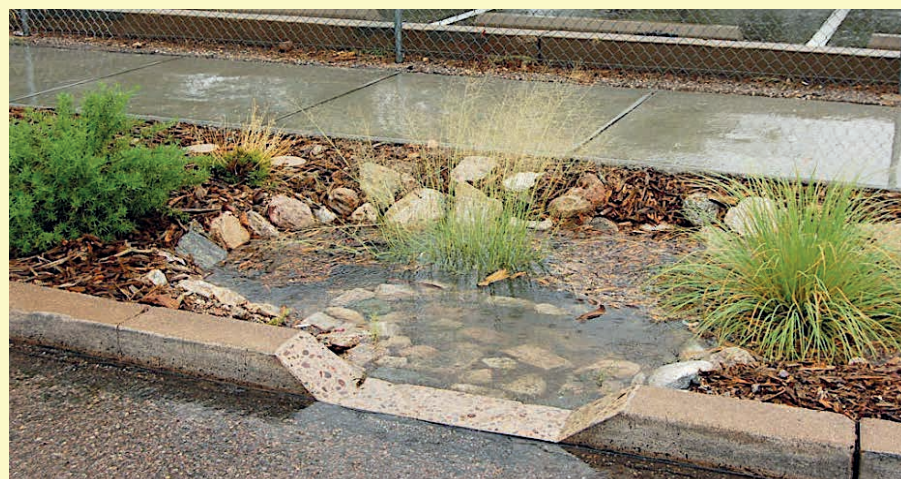
A curb cut allows water to run into a landscaped area between the sidewalk and the street.
