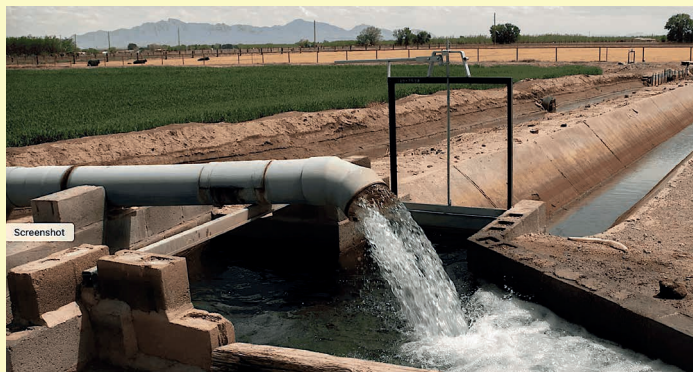
Middle Río Grande District irrigation
