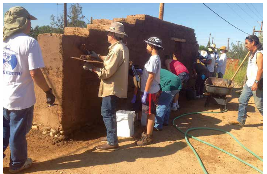
Top: Agua Frians making adobes for Gateway Monument, 2013. © Lois Mee Bottom: Agua Frians plastering Gateway Monument, 2015. © Lois Mee
