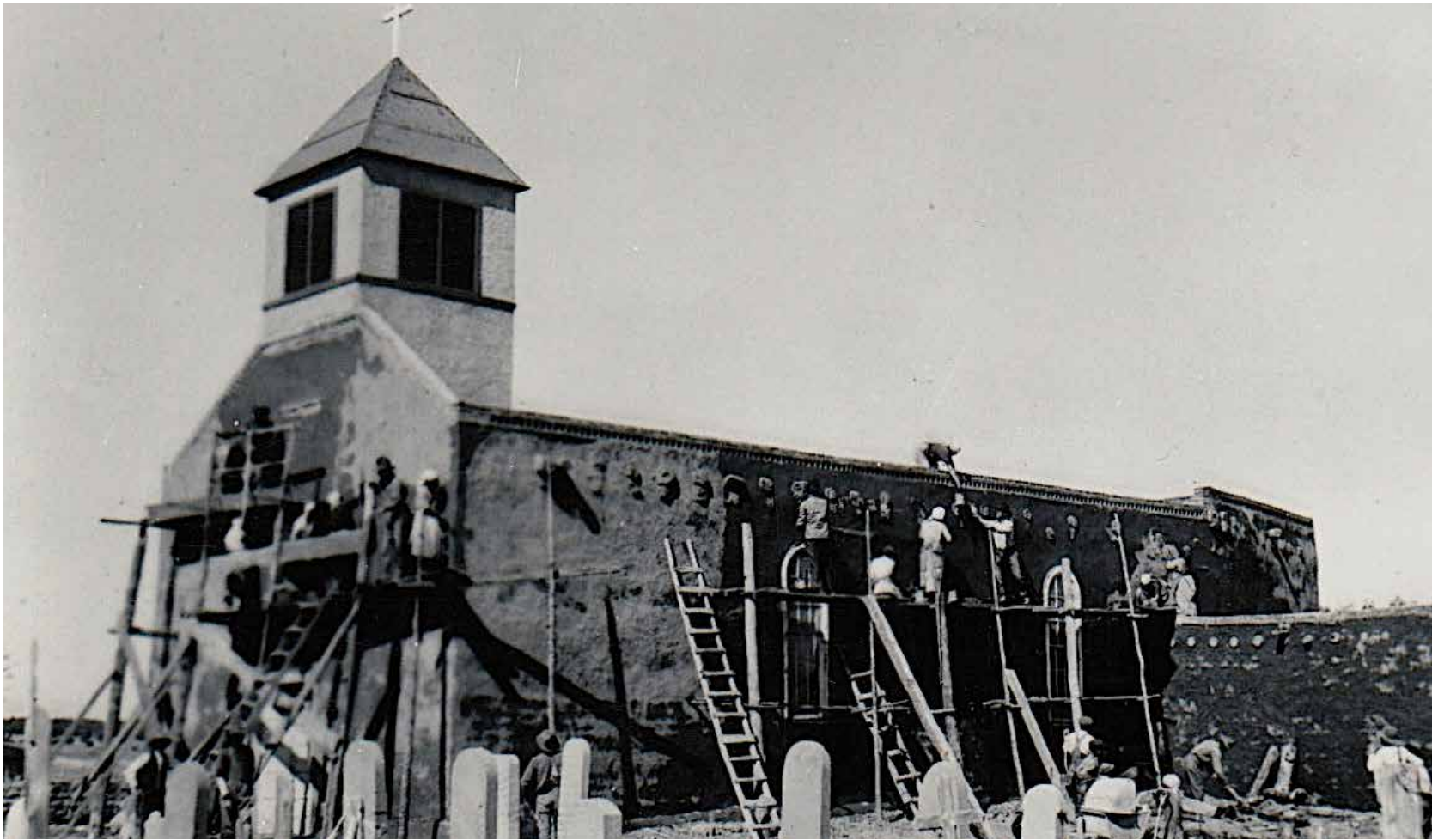
Mud plastering, San Isidro Church, Agua Fria; Museum of N.M. #005056 by T. Harmon Parkhurst, 1925
