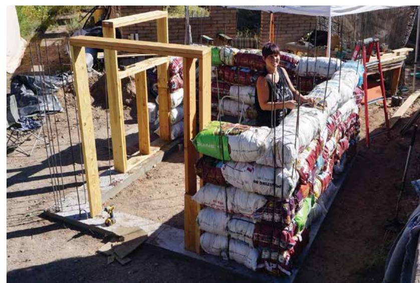
Constructing an Ubuntu-Blox shed north of Santa Fe
