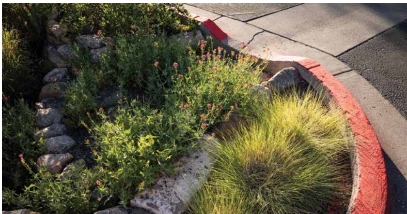
Baker's rain gardens collect rainwater from street runoff. It infiltrates through planted areas that naturally remove toxins, grow food for humans and wildlife, and reduce erosion downstream.
