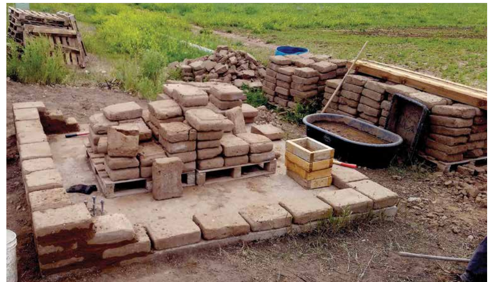
Adobe blocks and mortar
