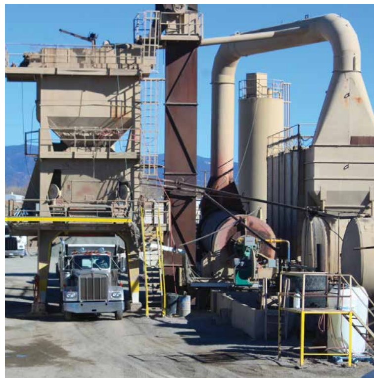
Associated Asphalt & Materials plant in Santa Fe, N.M.
